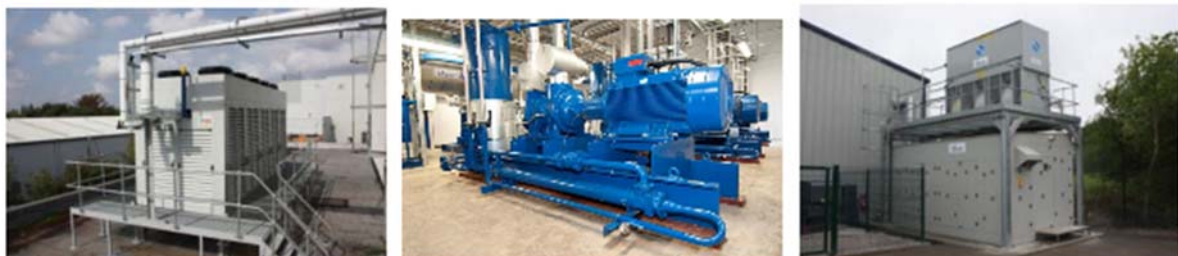
examples of packaged ammonia systems
